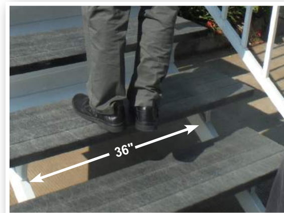
QuickStep stair treads shown with QuickStep stair stringers at 36" centers.
