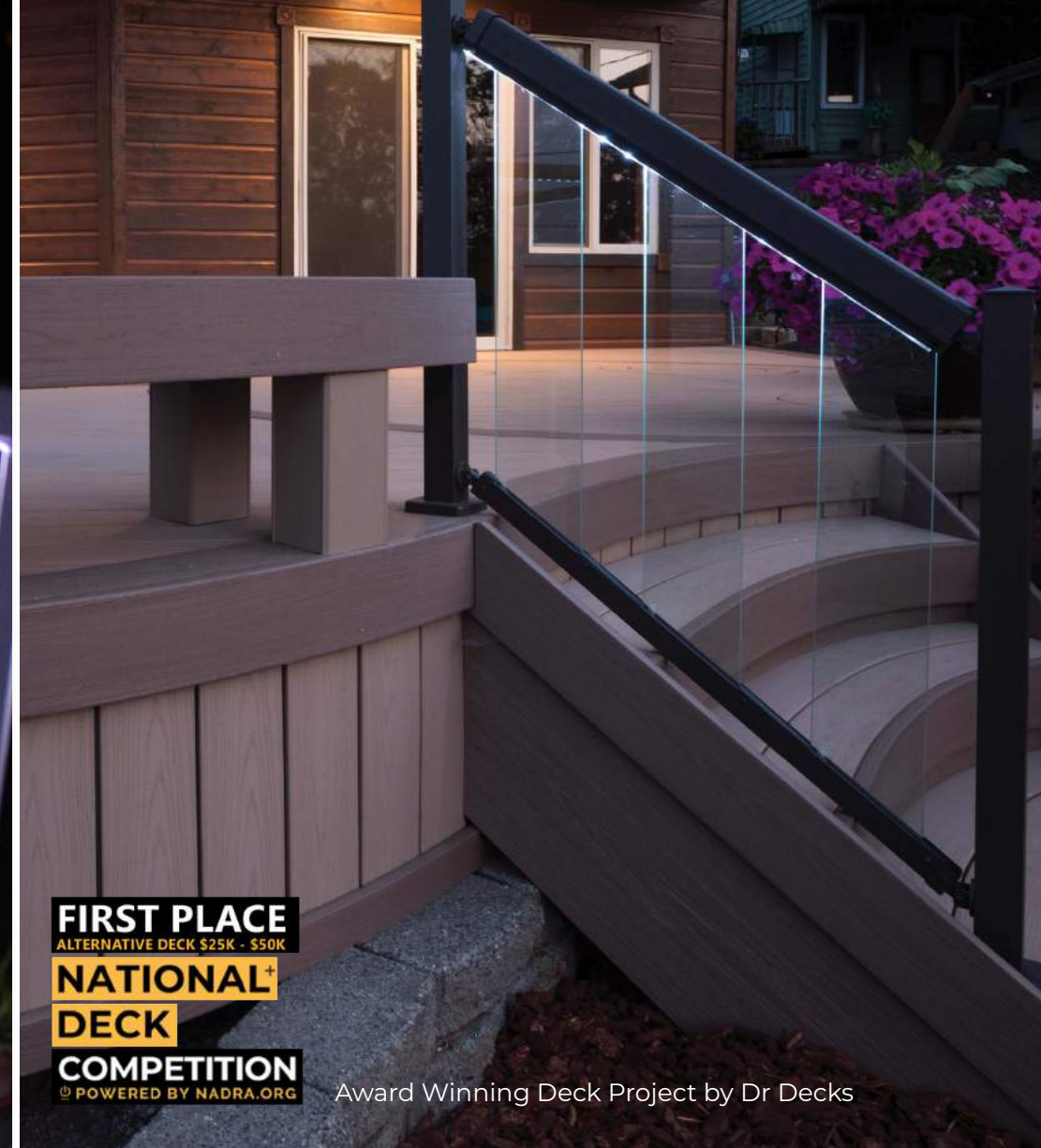
Yard Bronze Regal Aluminum Railing With Glass Stair Pickets.
