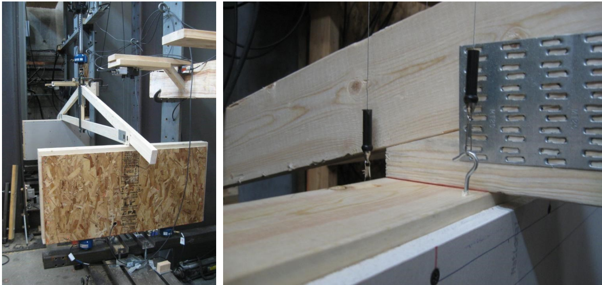
FIGURE 3. WALL CONSTRUCTION TEST SETUP
