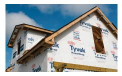
**SEAL THE BUILDING ENVELOPE** Facilitates an energy efficient building, suitable for use in residential and commercial application.
