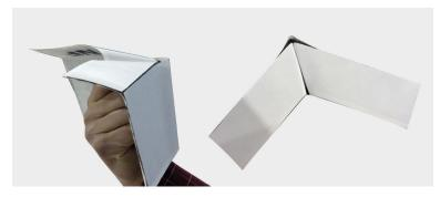
**A-7. Form Recessed Window Corner.** Remove narrow-width release paper and, using the creases made in Step A-6, carefully press together the exposed butyl within the corner fold to create Recessed Window Corner. Repeat with the 3 remaining 12" pieces of FlexWrap™ NF.
