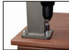
Fasten Post to Deck Surface
