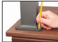
Mark and Pre-drill Holes
