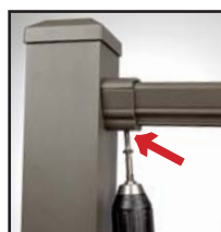
Fasten top rail to bracket
