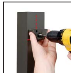
Center bracket and attach to post
