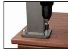
Fasten Post to Deck Surface
