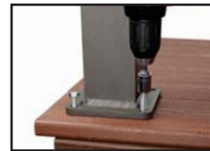
Fasten Post to Deck Surface
