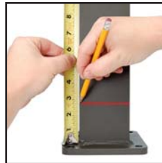
Measure up 2-1/2" from top of base plate
