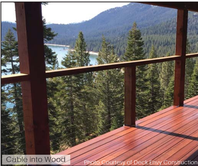
Cable into Wood
