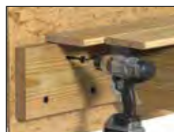
LEDGER BOARD CONNECTIONS
