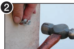
2 Carefully tap the Expansion Bolt until the machine threads protrude 3/4".
