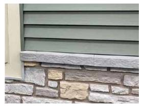
Architectural Sill Corners can be used as a corner or to terminate the end of a run.
