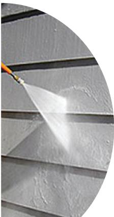
**Left:** Surfactants such as exterior siding cleaners used in pressure-washing can break down the resistance of a housewrap.
