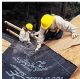
Roll out membrane; cut to required lengths. Extract RIPCORD following instructions above. Position membrane at start up area aligning center on valley. Remove one side of the release paper. Press membrane into place with hand smoothing outward towards edge. Repeat on other side of valley.
