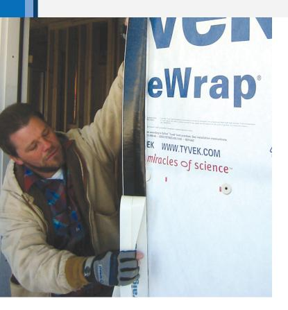
DuPont™ StraightFlash™ VF ties the window or door frame directly to the sheathing or water-resistive barrier to protect from bulk water leaks.
