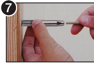
7 Insert cable all the way into Quick-Connect® fitting until it stops. Jaws will lock automatically.
