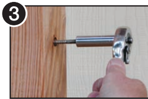
3 Drive Hanger Bolt into post using 7/16" socket or electric drill with 1/2" chuck.
