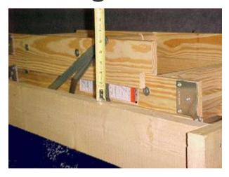
1. Measure how high the attic stairs are above the rough frame (2x6). This will determine the height of Attic Tent needed. Attic ladder side rail made with a (1x4) need a 7inch height Attic Tent.
