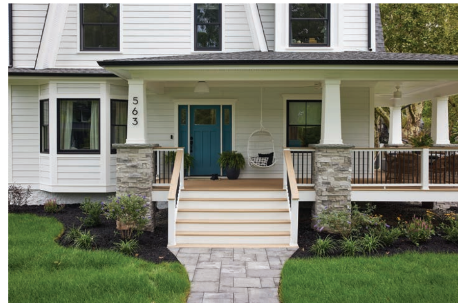
Weathered Teak® Porch + AZEK® White Trim Boards as Fascia and Risers + AZEK White Tapered Column Wraps
