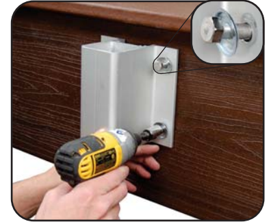
Step 2: Attach bracket to fascia
