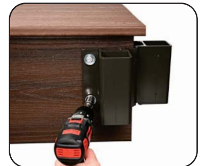
Step 2: Attach bracket to fascia
