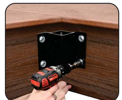
Step 2: Attach bracket to fascia
