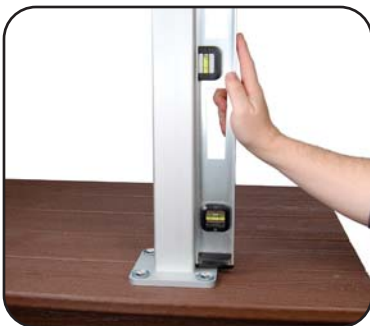
Step 4: Ensure post is plumb, adjust as needed. Tighten fasteners and ensure proper engagement into blocking.
