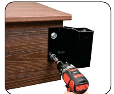
Step 2: Attach bracket to fascia
