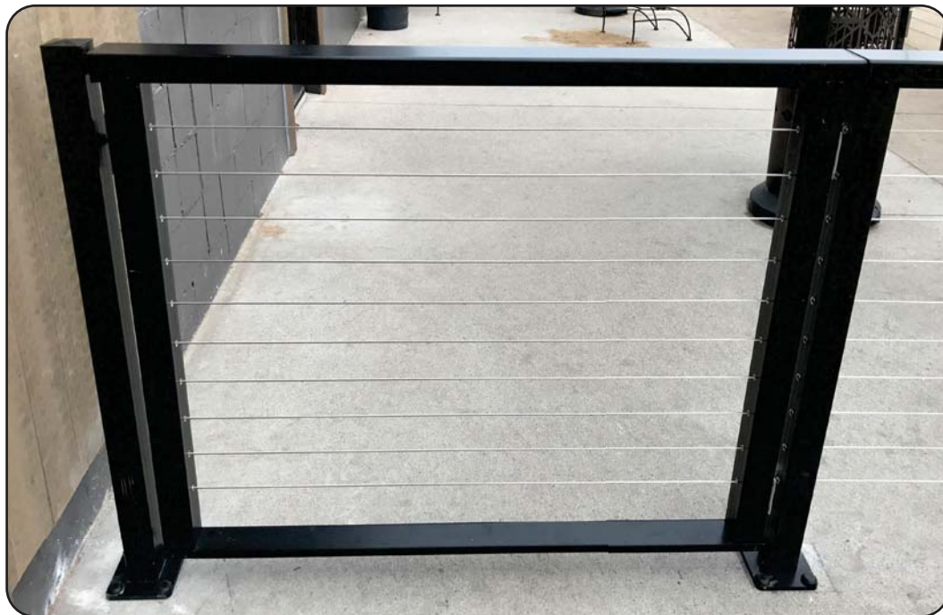
Completed Gate Assembly (Latch & Hinge on Opposite Side)
