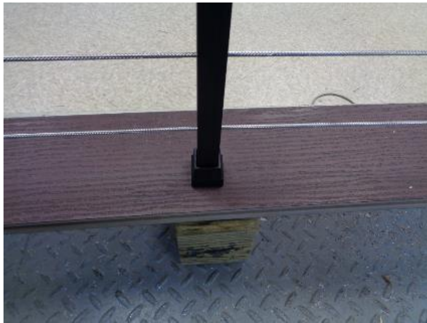
Photo No. 23 Intermediate Support Baluster Deck Board Socket Bracket
