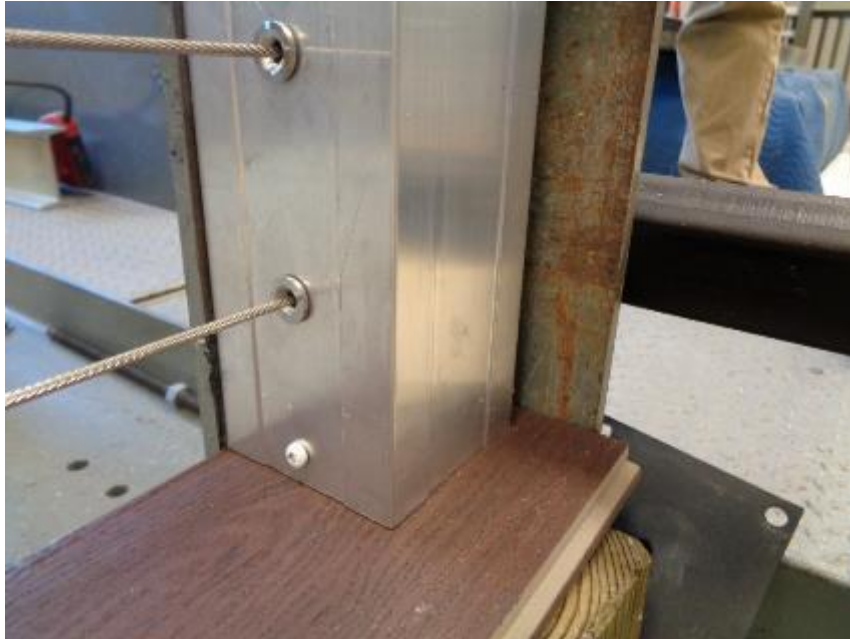
Photo No. 21 Horizontal Cable Rail Infill to Post Connection
