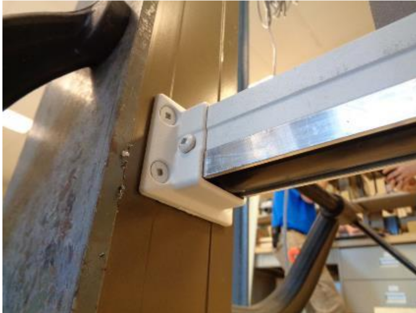
Photo No. 17 American, Arabian and Keystone Series - Bottom Rail Socket Bracket; Rail-Bracket-Post Connections
