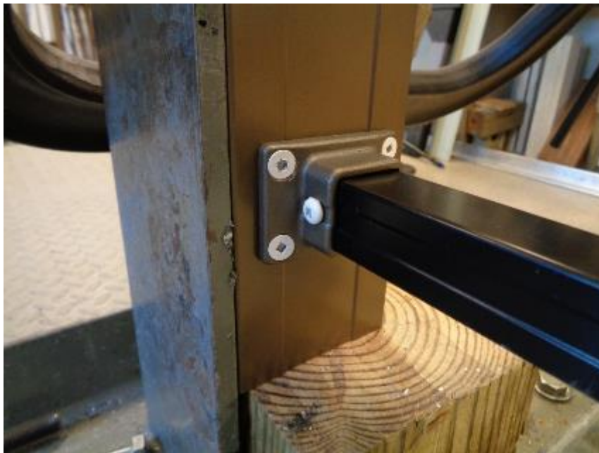
Photo No. 18 Outlook Series - Bottom Rail Socket Bracket; Rail-Bracket-Post Connections
