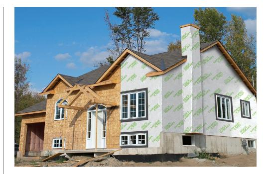
Vycor<sup>®</sup> enV-S<sup>™</sup> sheet-applied, fully-adhered weather resistive barrier provides exceptional protection against water damage and air infiltration. It helps preserve the home's structural integrity and contributes to improved energy efficiency.
