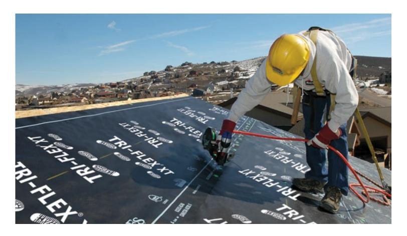
Tri-Flex® XT synthetic roofing underlayment is a high performance water-shedding underlayment. The new coating formulation provides superior foot traction. It is 20 times stronger than #30 felt and withstands high wind conditions; it is lighter than #30 felt and covers more area. The product is mechanically attached to the roof and can be used alone or in conjunction with GCP self-adhered underlayments.
