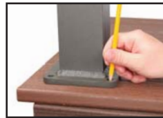
Mark and Pre-drill Holes
