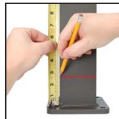
Measure up 2-1/2" from top of base plate
