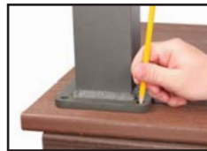
Mark and Pre-drill Holes
