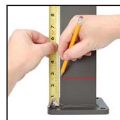
Measure up 2-3/8" from top of base plate
