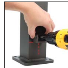
Center bracket and attach to post
