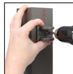
Center and fasten backer plate to post with arrow pointing right
