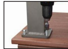
Fasten Post to Deck Surface
