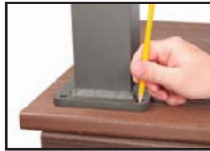
Mark and Pre-drill Holes
