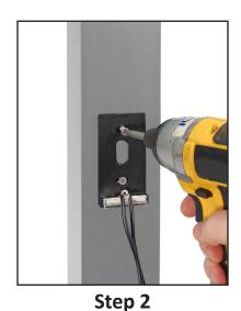
Locate and attach backer plate to post using 2 ea. self-drillng screws. Ensure light is plumb and centered
