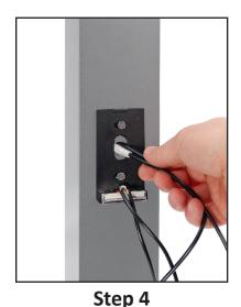
Pass wires through the hole and fish up the post to connect to perimeter wires. Use of a fish tape or similar item may be useful.
