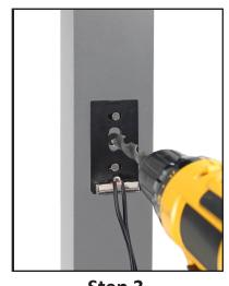
Step 3 Drill 1/2" diameter hole to allow for passage of Quick Connect wires. Clean metal shavings from fixure.
