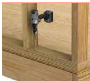
BOTTOM PLATE TO RIM BOARD
