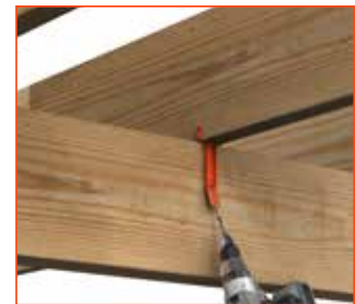
BEAM TO JOIST
