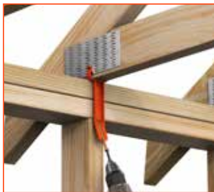
DOUBLE TOP PLATE TO TRUSS
