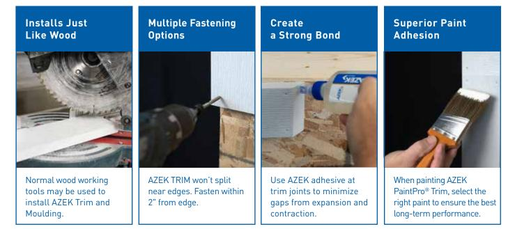
AZEK Trim and AZEK Mouldings should be installed using the same good building principles used to install wood trim and mouldings and in accordance with the local building codes and AZEK's complete installation guidelines that can be found at www.azekexteriors.com.
